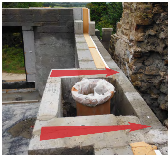
The arrows in this photograph show where a thermal bridge has been formed by the chimney structure which passes right through the insulation layer. Image courtesy of Gavin O'Shea
