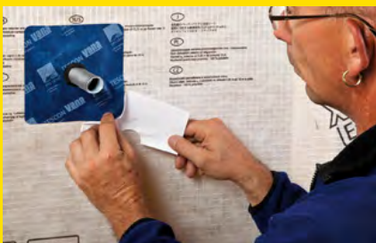
Airtightness gasket
