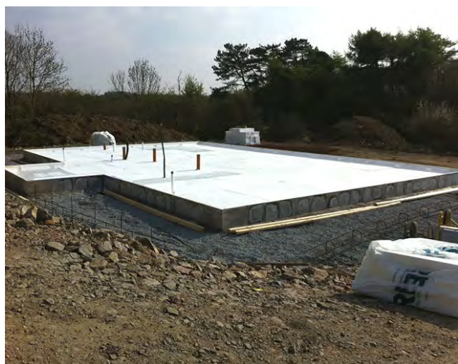
This load bearing insulated foundation system helps eliminate thermal bridging from foundations. Image courtesy Kore Systems
